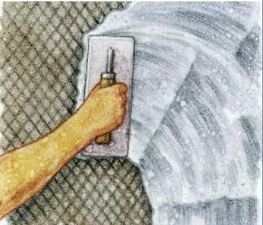
PREPARE THE SURFACE
