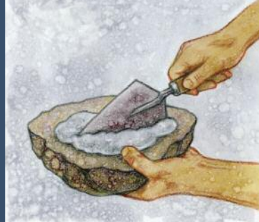
APPLY THE MORTAR
