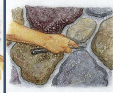
FINISH THE JOINTS
