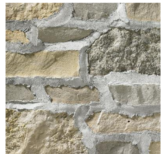
OVERGROUT JOINT
