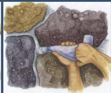
GROUT THE JOINTS
