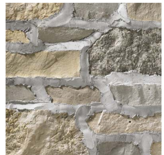
OVERGROUT JOINT
