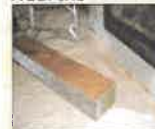
Wire Mesh applied over drywall.
