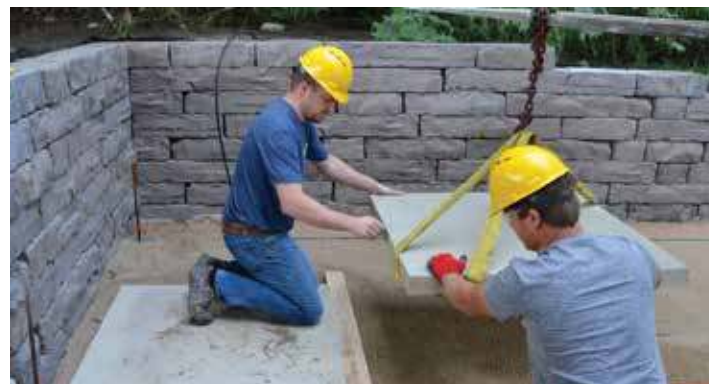
Set slabs with Miros lifting device or properly rated nylon straps
